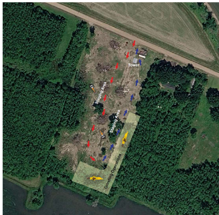
Church Point #1 – Site 3
