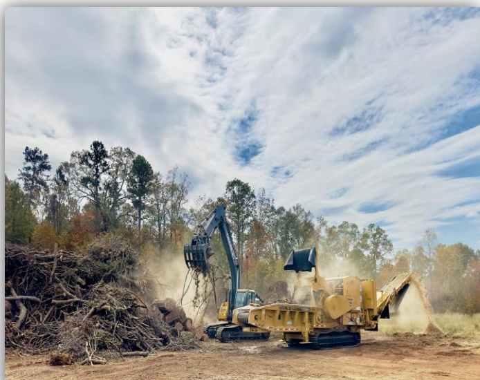
Grinding Debris to Reduce
