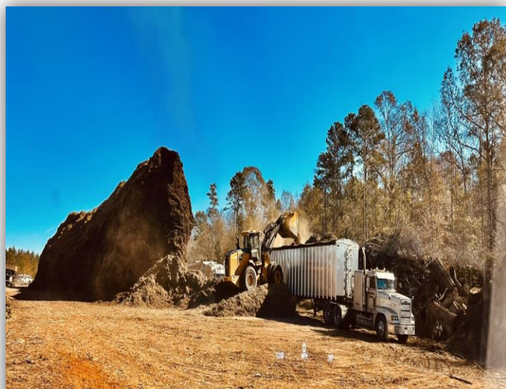
Final Haul Out of Reduced Debris
