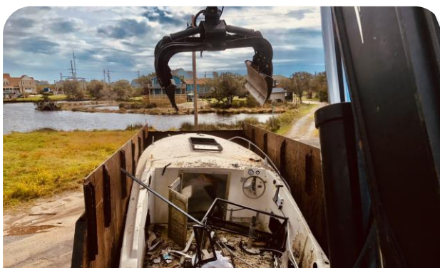
Waterway Vessel Removal
