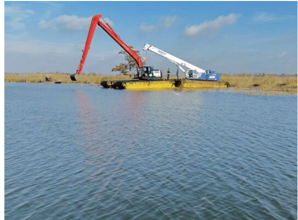
Amphibious excavator and crane recovering storm debris from open water.
