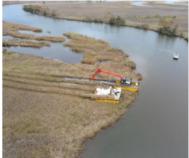
Amphibious/pontoon equipment minimizes wetland disturbance during access and recovery.
