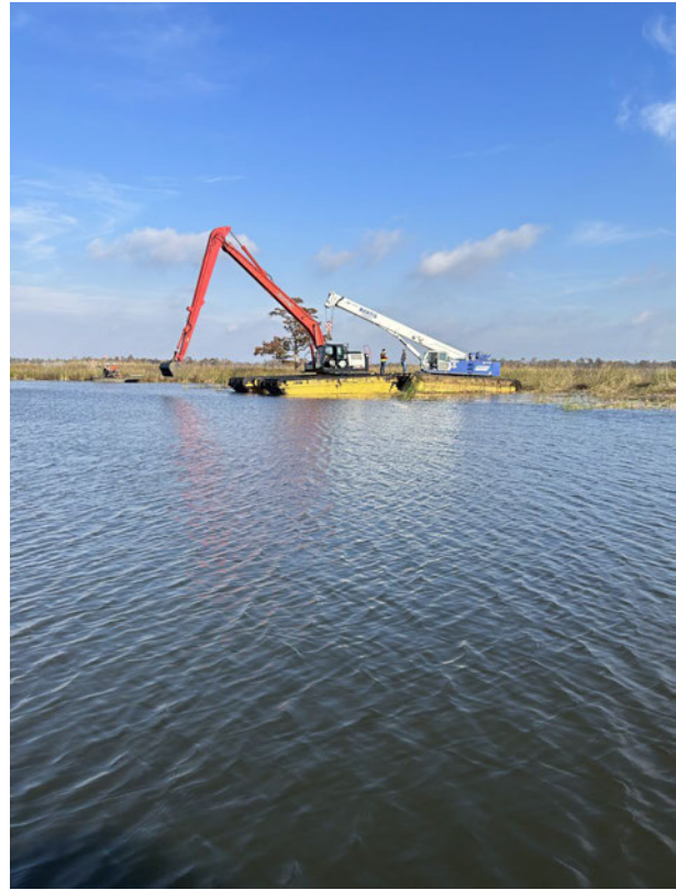
Barge-mounted crane removing heavy/large debris from a navigable reach.
