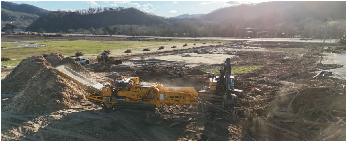
Horizontal grinding of vegetative debris at a WDS-operated reduction site (fire watch maintained).
