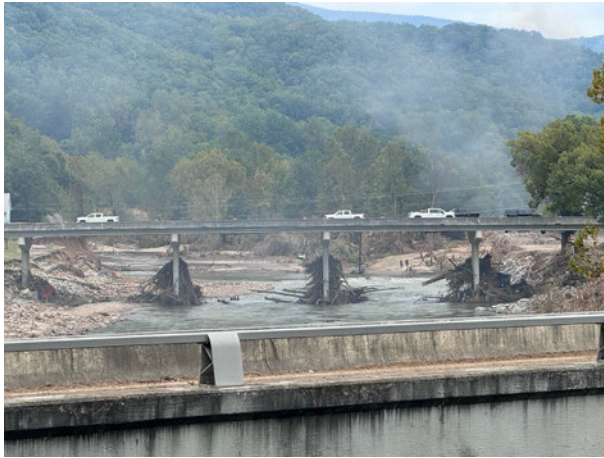
Debris removal at a drainage control structure — restoring designed flow capacity.
