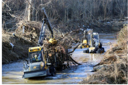
Twin amphibious excavators clearing a debris-choked channel.
